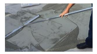
Spread DRiBOND® with the ST300 Roller Screed Tool at the recommended thickness of 3/8". For uneven surfaces or dips, consider increasing the screeded thickness to a maximum 1" to level out the surface. Do not compact your screeded DRiBOND®.
