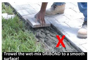
Wet set the border pavers using a ½" notch trowel with a wet mix of DRiBOND® to create a water retention border. There should be no air pockets or voids under the wet-set border tiles.
