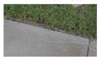
Cut two or three grooves into the existing concrete slab at the border. This enhances bond strength when border pavers are installed.
