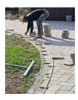
Leave a border width of one full border paver from each edge to lay the wet set border pavers. Extend all overlaid hardscape material over the border paver edge distance from each edge. All hardscape material placed within the zone of a border paver will be cut and removed to allow the border paver material to be wet set. As per the above right picture, sections of PVC pipe can be connected to mark a radius cut line.
