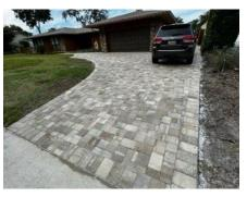
Tie the pavers into the street surface and other areas such as sidewalks by creating a transition area where necessary to avoid a tripping hazard.
