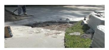
Once damaged concrete is removed, cut V-shaped notches into the existing concrete substrate using a wet saw and diamond blade. This will help tie-in the new concrete to the existing concrete.
