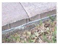
Remove any excess product from the edge of the finished paved area. The above photo shows a proper border paver installation.
