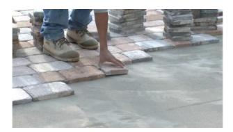
Without walking on DRiBOND®, lay pavers square to the structure or create a right angle to start the field according to the selected pattern.
