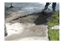
Next, fill the removed area with 6,000 psi fast set concrete. Completely fill in the notches that were cut in the existing concrete and allow the newly laid concrete to cure.
