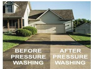
Remove stains and oil spots with appropriate stain removers and degreasers. Power wash the concrete surface to remove any dirt from the area to be covered. It is important to apply DRiBOND° over a clean dry surface. Be sure to let the surface dry completely before applying DRiBOND°.
