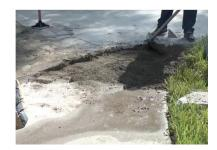
Next, fill the removed area with 6,000 psi fast set concrete. Completely fill in the notches that were cut in the existing concrete and allow the newly laid concrete to cure.
