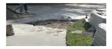
Once damaged concrete is removed, cut V-shaped notches into the existing concrete substrate using a wet saw and diamond blade. This will help tie-in the new concrete to the existing concrete.
