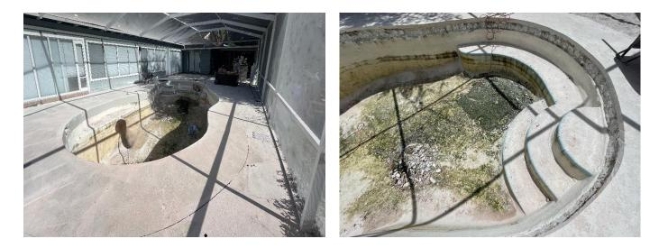
Remove stains and oil spots with appropriate stain removers and degreasers. Power wash the concrete surface to remove any dirt from the area to be covered. It is important to apply DRiBOND<sup>®</sup>over a clean dry surface. Be sure to let the surface dry completely before applying DRiBOND<sup>®</sup>.
