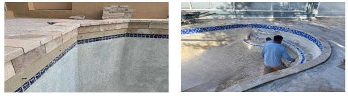
We recommend completion of all coping and waterline tile work prior starting your DRiBOND<sup>®</sup> pool deck overlay. Starting with interior pool and pool edge work allows work site access without stepping on screeded DRiBOND<sup>®</sup>. Install coping using a wet mix of DRiBOND<sup>®</sup> to ensure proper edge setting prior to ANY watering of overlaid pool deck material.
