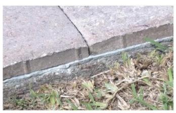
Remove any excess product from the edge of the finished paved area. The above photo shows a proper border paver installation.
