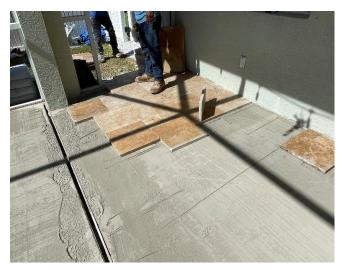
Without heavily walking on the DRiBOND, lay your hardscape paver square to the structure or coping edge and start to lay the field according to the selected pattern. Always maintain appropriate pitch toward drain(s).
